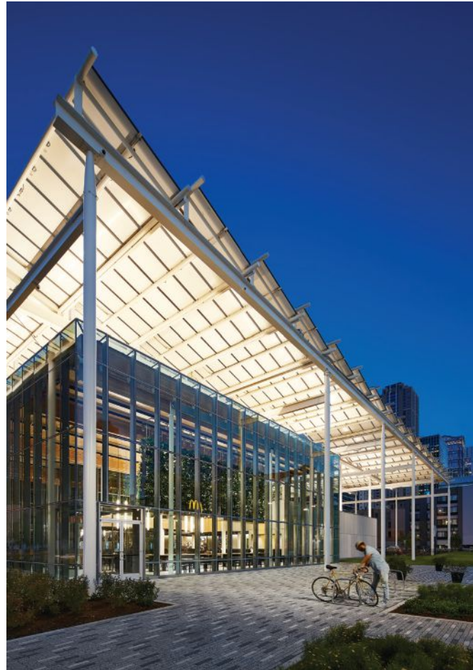
Solar panels generate 60 percent of the building's energy
