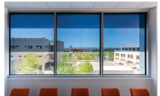
In-pane zoning on display at the University of New Mexico Farris Engineering Center.
