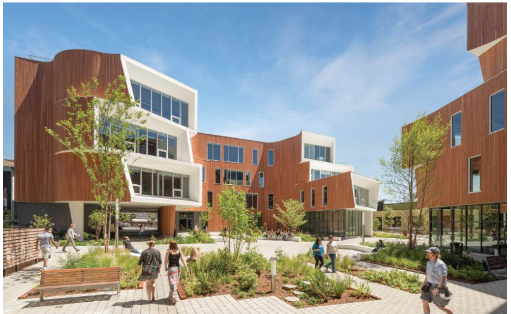
Although the owner did not pursue LEED certification, “my guess is One North would probably exceed LEED and Passive House standards,” says project architect Kevin Valk. Courtesy of Holst Architecture | Photo: Andrew Pogue
