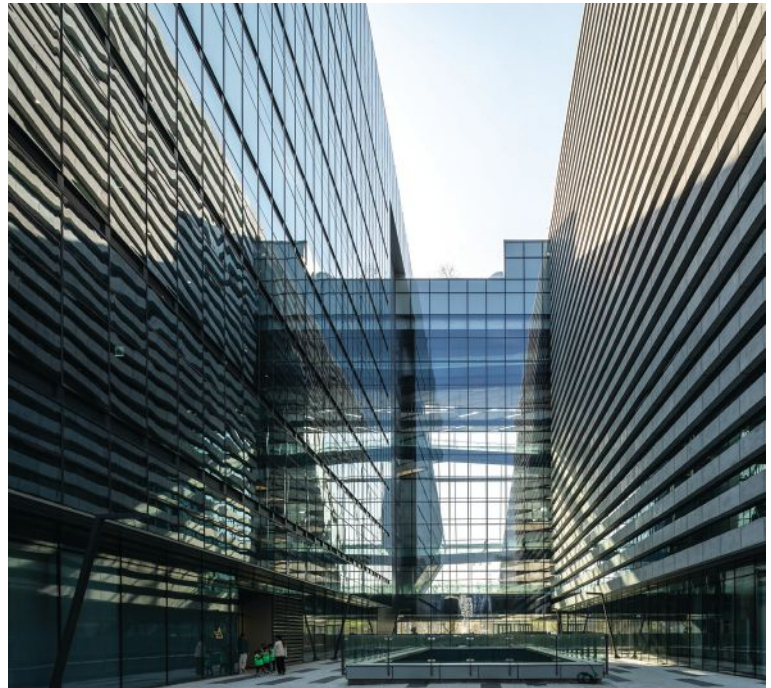
Central open-air courtyard, looking west through full-height atrium
