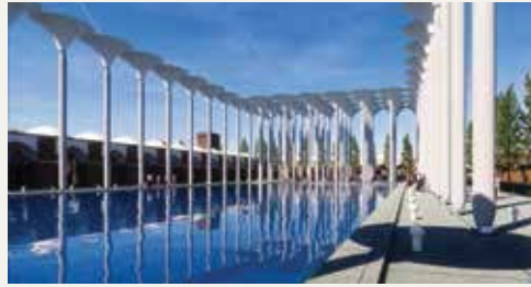
Regeneration of Risbaf Industrial Heritage Cultural Entertainment Commercial Complex, Isfahan, 2018
