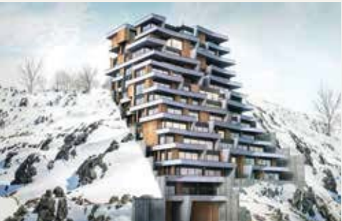
The Terrace, Darbandsar, Under Construction
