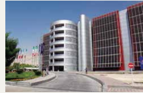
South Pars Gas Company, Asalooyeh 2005-2014
