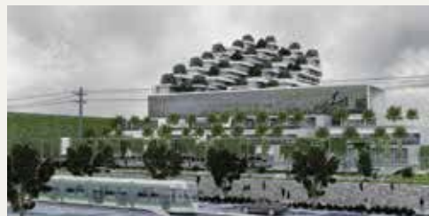
Plasco commercial Complex Rebuild Tehran
