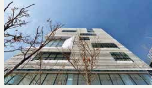
White Office Building, Tehran 2015
