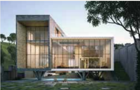
Fasham Villa, Fasham, Under Construction
